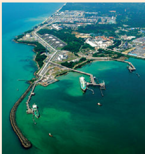
PETRONAS Integrated LNG Complex in Bintulu is still one of the world's largest of such facility at a single site.
