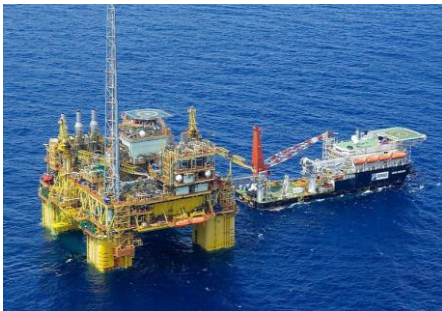
Gumusut-Kakap production facilities, Shell's first deepwater project in Malaysia
