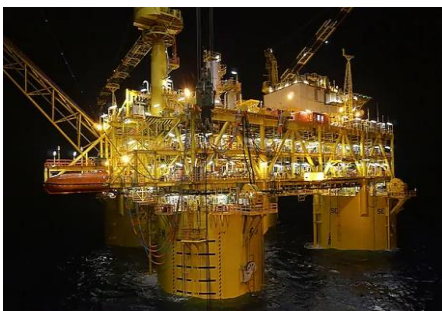
Shell's Malikai deepwater facilities, the first tension leg platform in Malaysia
