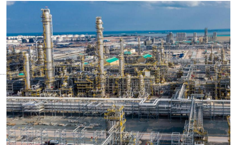
Pengerang Integrated Complex, Johor
